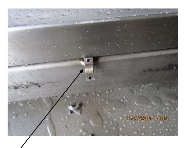
• CUT OFF WELDED SPLIT COLLAR BRACKET & GRIND SMOOTH.
