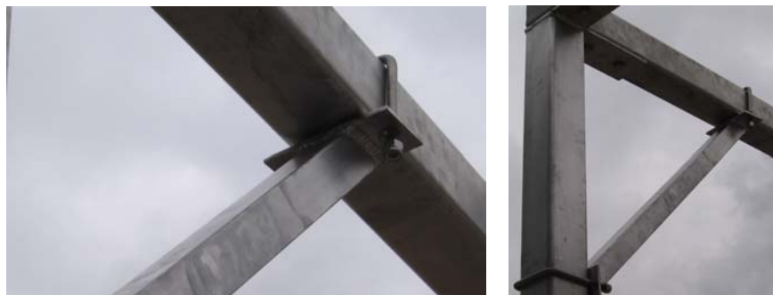
Figure 1-3. Mounted Post-to-Header Gusset
