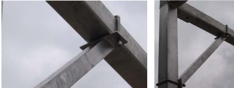
Figure 3-3. Mounted Post-to-Header Gusset
