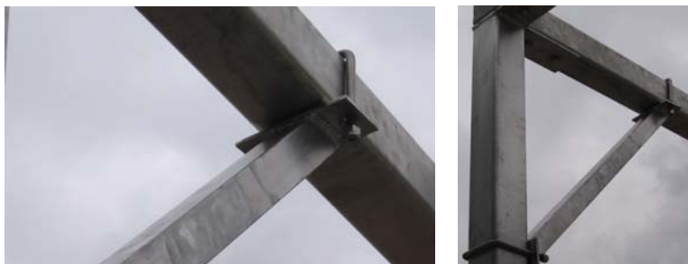
Figure 1-3. Mounted Post-to-Header Gusset
