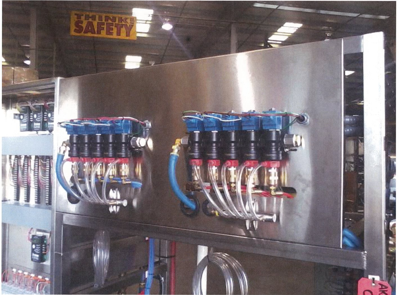
Panel board for DSI with Hydraflex Solenoids for soap and wax
