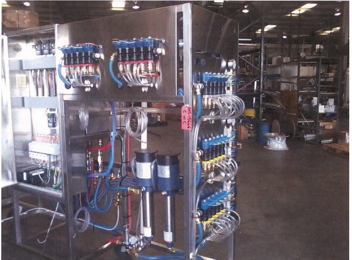
Picture of DSI chemical injection system with HydraFlex solenoids and injectors The top of the board shows the high pressure soap and Wax The right hand side shows the low pressure functions for Tire Cleaner, Foam Brush and Low pressure wax or triple foam.
