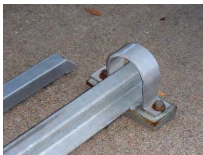
End of Track Stop
