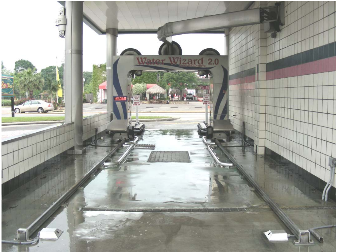
Water Wizard 2.0 Typical Installation
